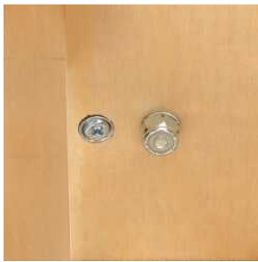
Micro-Adjustment Screw for precise door alignment
