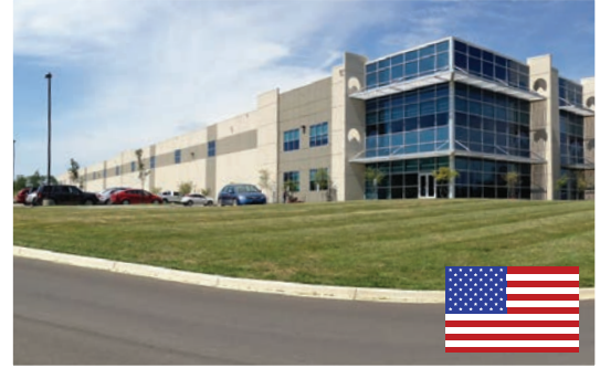
Made in the USA at Tresco's manufacturing facility in Louisville, KY
